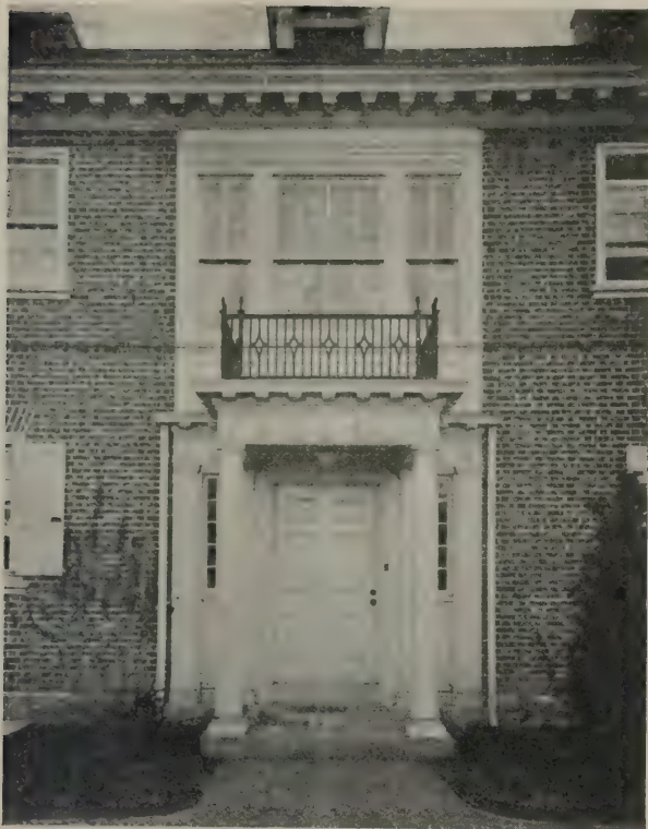
Fig. 3. Detail of House of George S. Robbins, Haverford, Pa.—D. Knickerbacker Boyd, Architect
